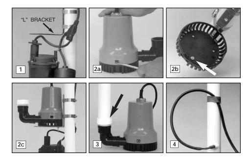
possible to avoid the return of discharged water to the sump. Be sure to seal the hole in the wall where the pipe exits and cement or clamp all connections securely to prevent leaking. No check valve is needed with this method of installation, as long as you use less than 20 feet of pipe.
